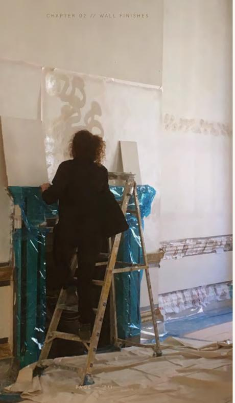
Rag Arts made samples for the mineral plaster using SOL silicate paint (Keim 'Optil') to which we added, marble dust, quartz and clay powder.
