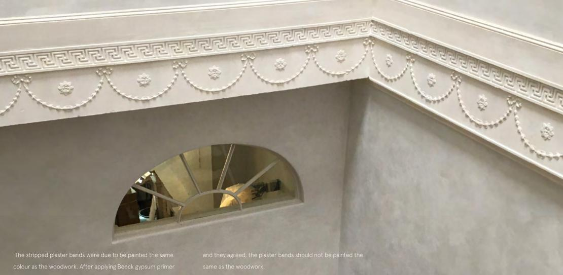
The stripped plaster bands were due to be painted the same colour as the woodwork. After applying Beeck gypsum primer and stain blocking any yellow stains with keim stain blocker, we realised that the plaster bands looked fantastic painted a chalky white
